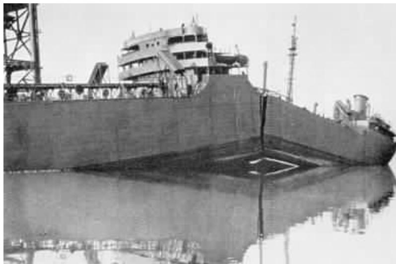
*Figure 2.7: Catastrophic failure of a Liberty Ship hull during the WWII era (Sanford, 2003).*
