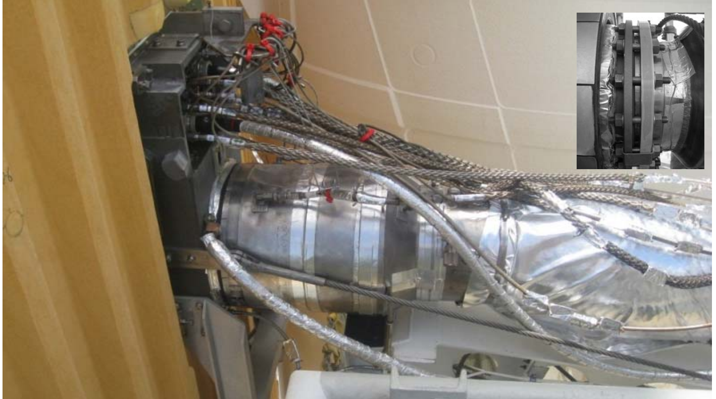
Figure 1: Flexhose assembly of ground umbilical carrier plate (GUCP) with and (inset) without weather-resistant shroud.
